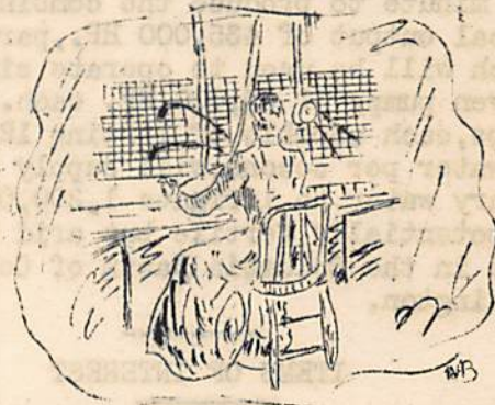
A Western Electric switchboard of the early '80s.
